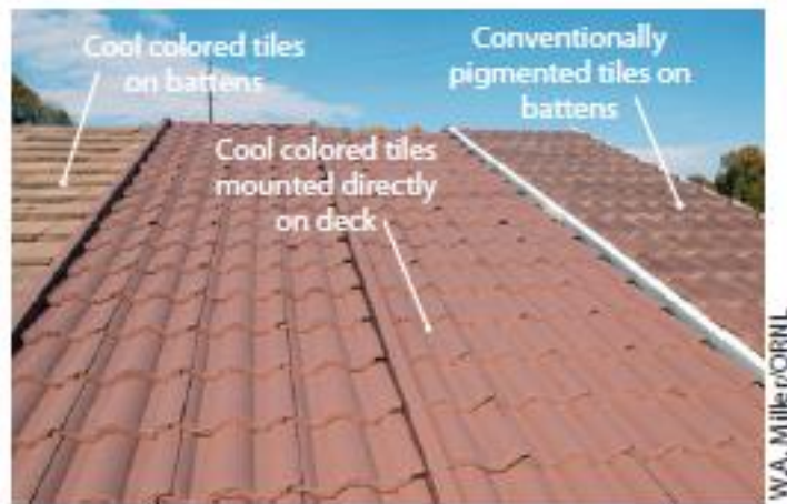
Figure 2. Conventional and Cool Colored Tiles (EPA 2011)
