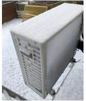
Figure 25: A Sanden CO2 heat pump water heater compressor working outside in 5°F (-15°C) weather.<sup>84</sup>
