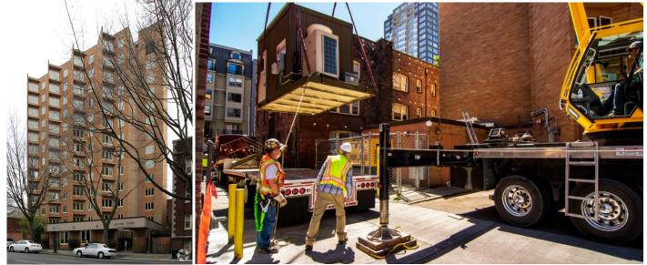
Figure 19: Bayview Tower in Seattle (left)<sup>55</sup> and the Origin heat pump water heater skid system being installed (right)<sup>56</sup>.
