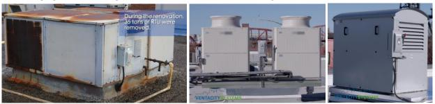
Figure 5: The before and after HVAC system of a Law Office retrofit in Portland Oregon. Old rooftop units (43 tons of heating) were replaced (left) with four heat recovery ventilators (right) and a variable refrigerant flow system (center) (18 tons of heating), reducing the buildings heating demand by 50%.<sup>27</sup>
