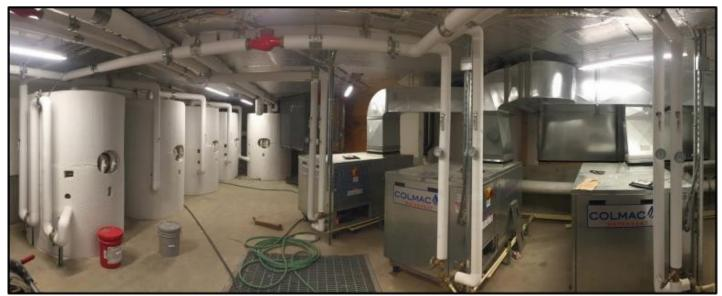
Figure 23: Ecotope Case Study "RCC" system for 194-unit Multifamily building, using best practices in central heat pumps for domestic hot water, from ACEEE presentation by Shawn Oram.<sup>1</sup>
