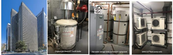
Figure 18: Arthur Erickson Place (left)<sup>52</sup>, the original gas-fired hot water boiler (center left), and the electrified heat pump water heater plant storage tanks (center right) and CO2 heat pumps (right).
