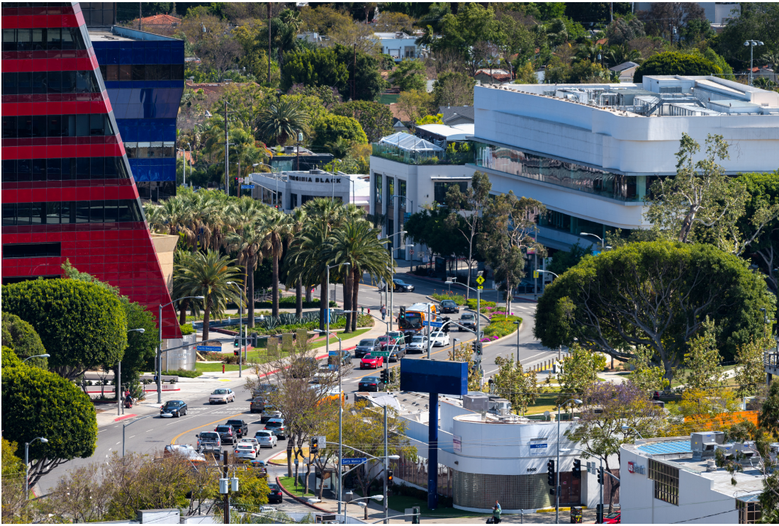
WeHo’s LEED Gold-certified Public Library with a rooftop solar array.
